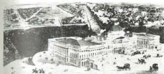
THE CAPITOL IN 1842 WITH COMPLETED WINGS - OLD DOME
