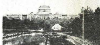
THE CAPITOL IN 1860 - NEW DOME UNDER CONSTRUCTION
